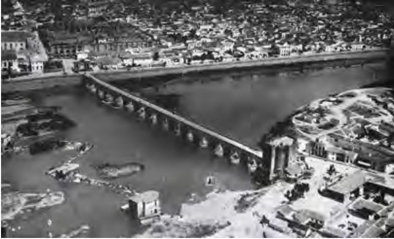
Fig. 1. Aerial view of the River Guadalquivir and the Roman Bridge. (From É. Lévi-Provençal, Histoire de l'Espagne musulmane , vol. I, Paris-Leiden 1950, Pl. V)
